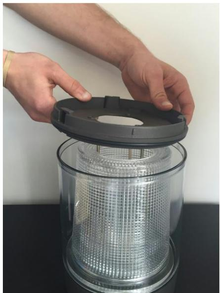
7.) Refasten the nuts to the three thin bolts, securing the bollard head mounting plate to the bollard head.
